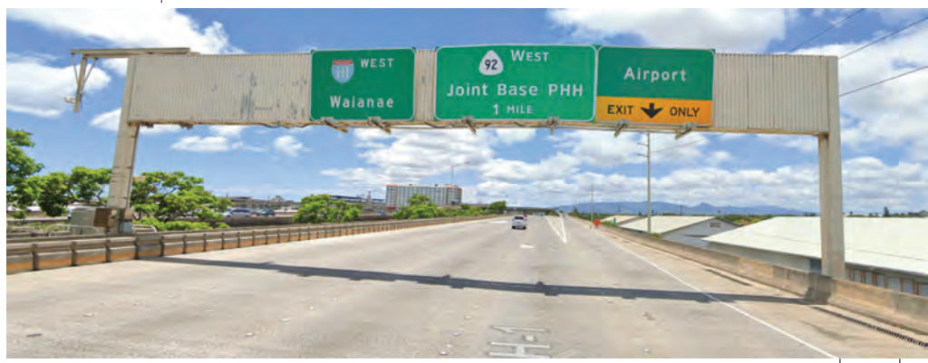
EXISTING SIGN STRUCTURE HIWB-505
