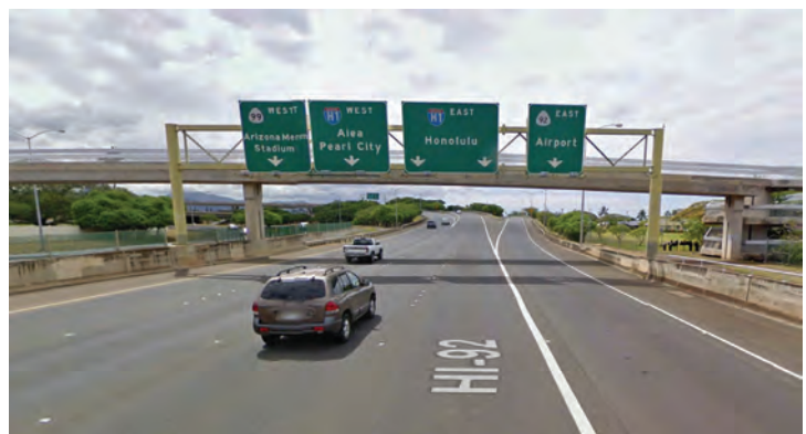
EXISTING SIGN STRUCTURE HIEBR-253
