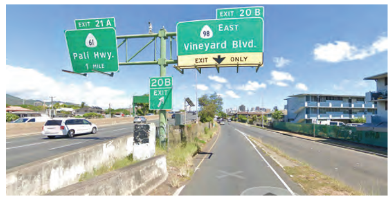
EXISTING SIGN STRUCTURE HIEB-305
