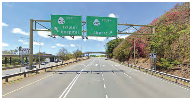
EXISTING SIGN STRUCTURE 78EBR-830
